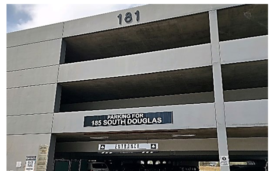
*Entrance to Student Overflow Parking at 181 S. Douglas St., El Segundo.
